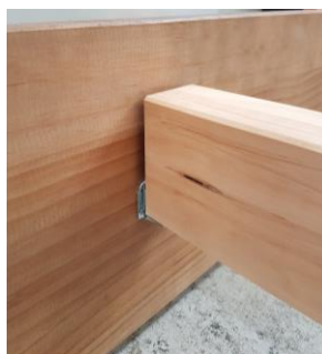
Centre Rail in place
